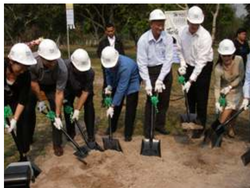
2009 Ground-breaking Ceremony, Photo courtesy HFHI
