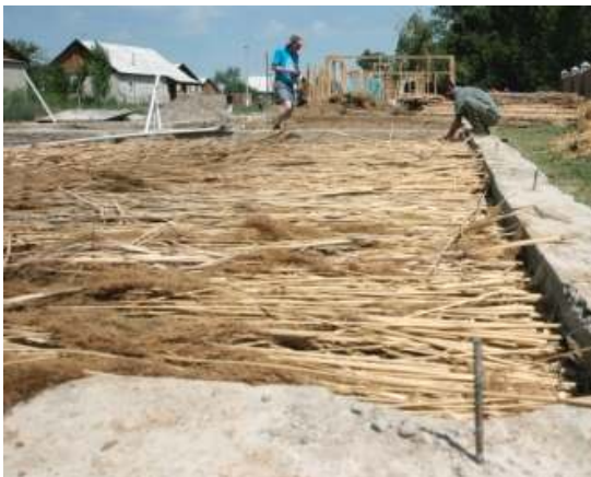
Volunteers backfill the ground under the floor construction with cane reeds.
