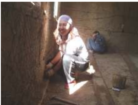
wood strips A Japanese volunteer installing wire net
